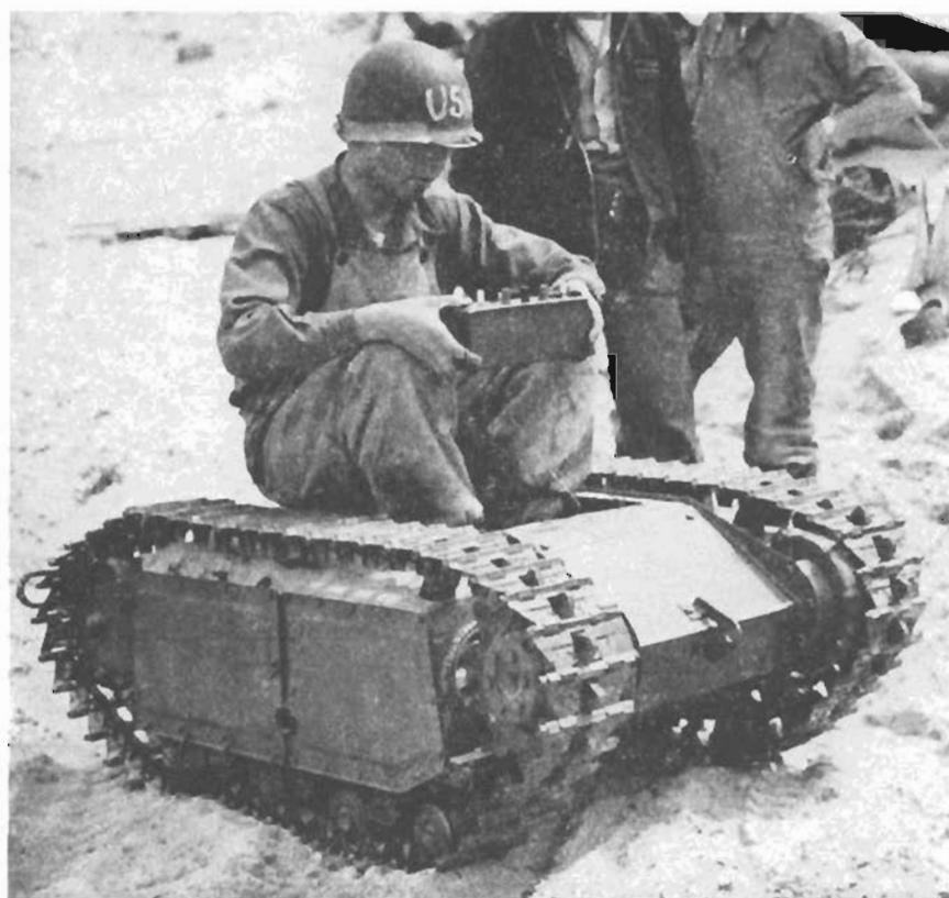
The Goliath (SdKfz 302) was solely remote-controlled with a 60kg charge. (US Army)
