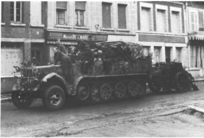
An m.Zgkw 8t. (SdKfz 7) eight-tonne medium prime-mover followed by the one-tonne le.Zgkw 1t (SdKfz 10). (Bundesarchiv)
