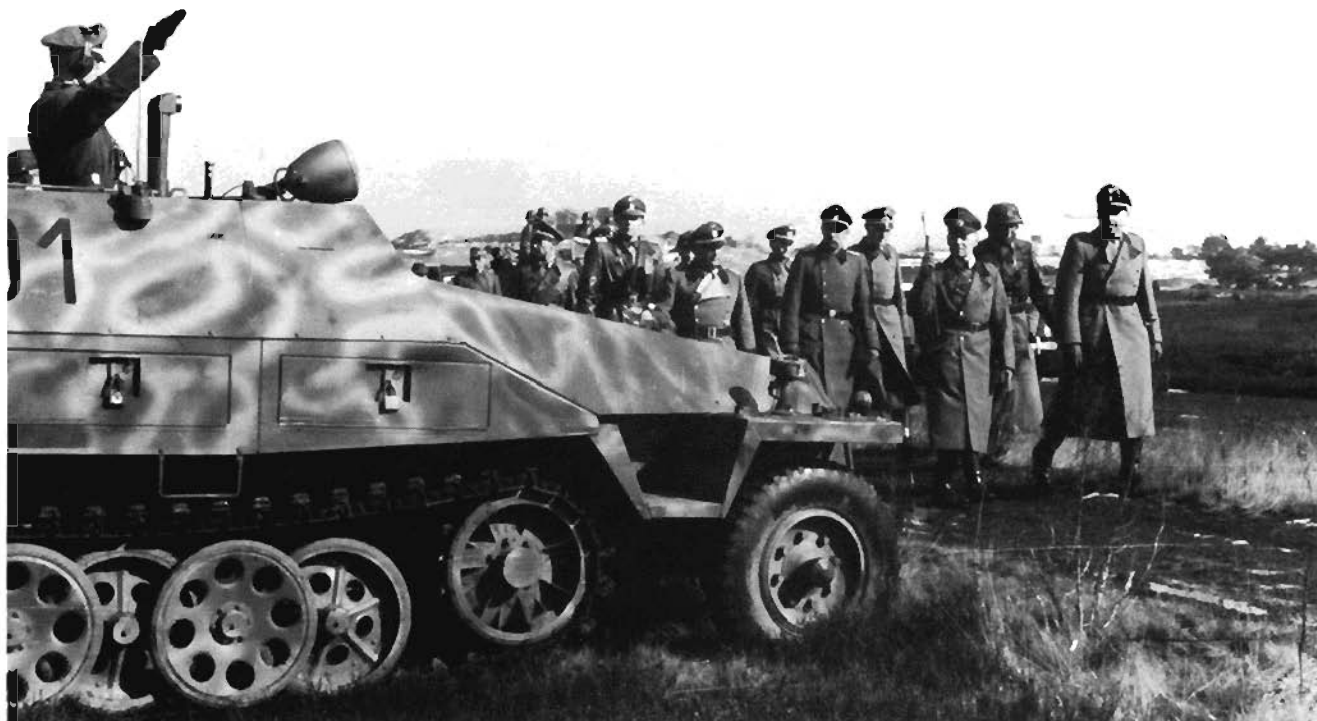
Above: Another version of the SPW was the SdKfz 251/15 — a specialised vehicle for artillery flash spotting. This one from the 12. SS-Panzer Division Hitlerjugend is being inspected by Generalfeldmarschall Gerd von Rundstedt (saluting with baton), commander of OB West — i.e. the Western Front. On his left is SS-Oberführer (later Brigadeführer) Fritz Witt,
