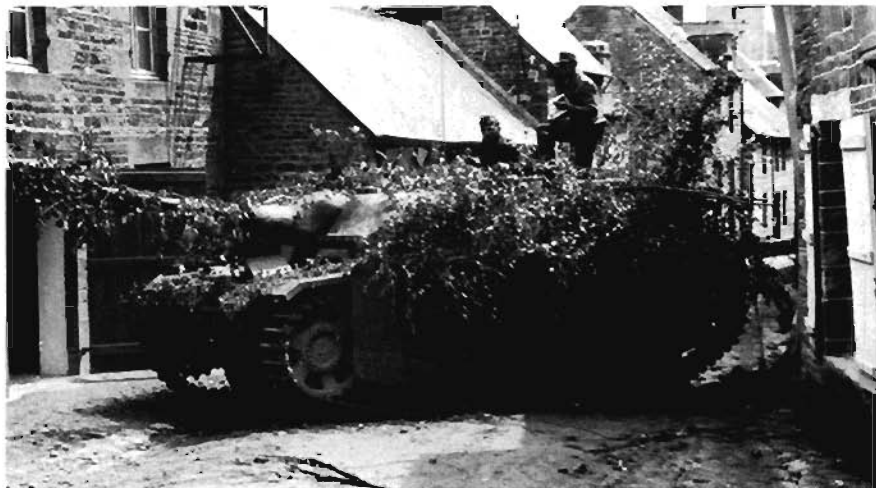
A StuG III of a Panzerjäger battalion of an army panzer division. Note the peculiar scolloped skirts of this Ausf G. (Bundesarchiv)
